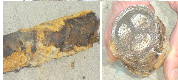
Fig. 12. Deterioration of underground power cables caused by stray currents
