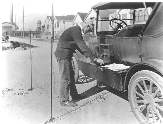
Fig. 3. Mobile laboratory built for determining dispersion of “stray” currents
