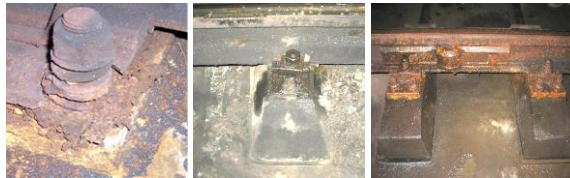
Fig. 9. Deterioration of the running routes rail fixings caused by stray currents
