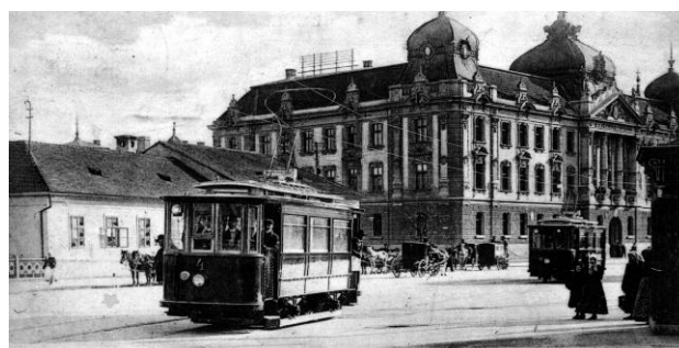
Fig. 1. First trams in Oradea city (traction with the help of two 35 kW engines)
