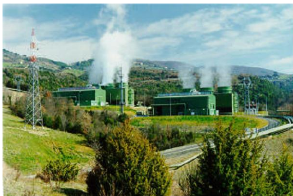
Fig.3. Geothermal power plant at Larderello today (courtesy of ENEL).
