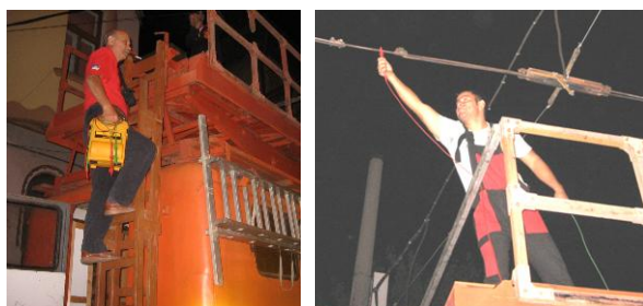
Fig. 1. Measuring the insulation resistance of the contact lines
