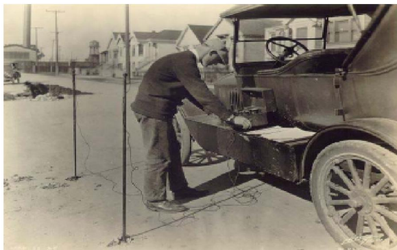
Figure 15. Mobile auto-laboratory designed for stray currents monitoring (Los Angeles 1910).
