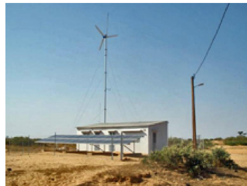
Figure 2: Solar wind Diesel hybrid power system for small village
