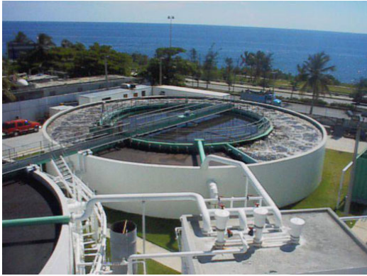
Fig. 5 - Fixed film treatment system.[9].
