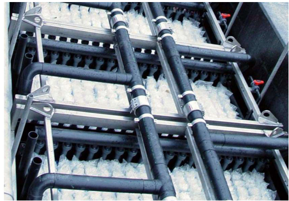
Fig. 6 - Membrane bioreactor treatment system[10].
