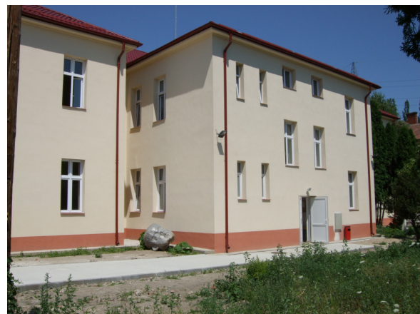
Fig. 3 - Demo-site building - main facade
