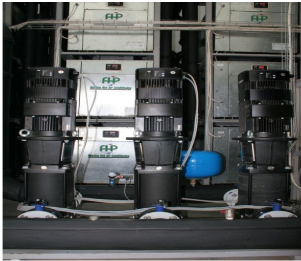
Fig.4. Heat pumps build in racks
