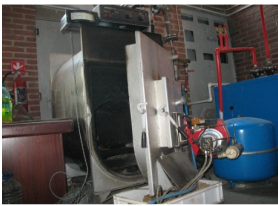
Fig. 4.1 55 kW PIFATI boiler- front view
