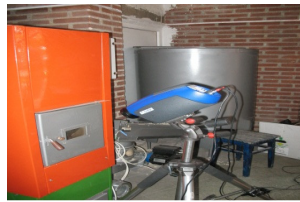
Fig. 4.2 30kW ERPEK boiler- front view
