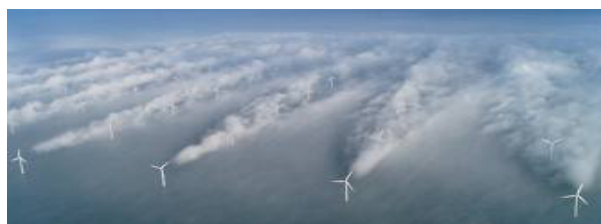
Fig. 1. Schematic representation of wake effect for wind turbine
