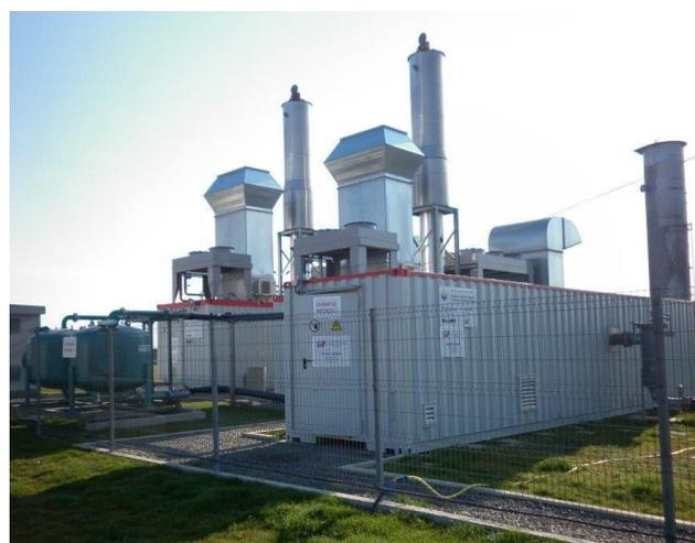
**Fig. 1 Landfill gas recovery facility, Chiajna [10]**
