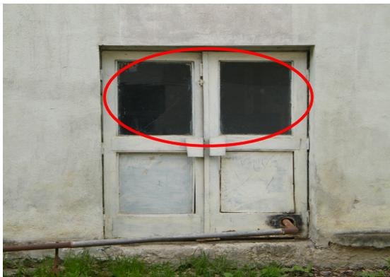
**Fig. 5 - Doors outer side of the block (the right in the direction of access in the block) presents metal sheet instead of glass - red marked area [12]**
