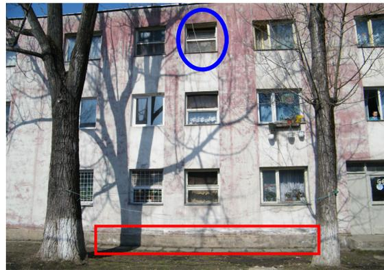
**Fig. 3 - Infiltration of water in the opaque elements of the tire of the building at the end of the lower bound - red border (ground level -building socket) and exterior joinery damaged (blue box) [12]**
