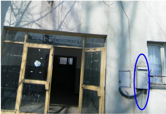
**Fig. 4 - The access exterior doors in the block are from metal with large glass surfaces [12]**
