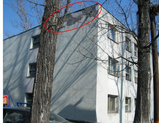
**Fig. 2 - Seeping water in the opaque elements of the building tire at the end of the superior (terrace level - top floor) [12]**
