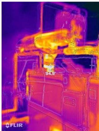
Fig. 11 – The path of the flue gases
